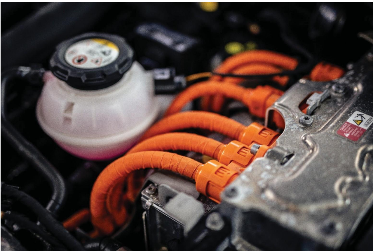
Cables with high voltage will most often be orange, as here in the engine compartment Photo: The Danish Emergency Management Agency
